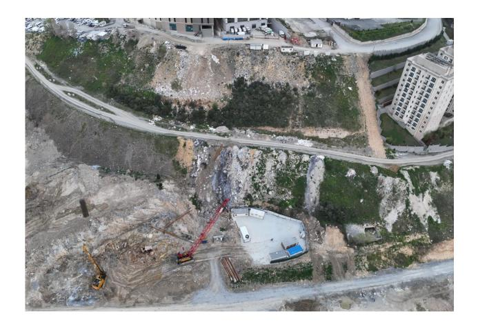
Picture 55 Building site pile foundation construction
